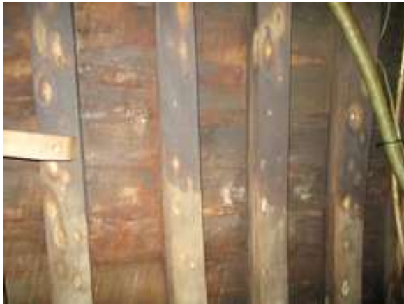
Interior view of frames and planks
